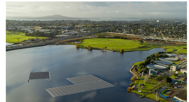
Vector PowerSmart 1 MW Solar Array - delivered for WaterCare at Rosedale treatment plant, 2020
